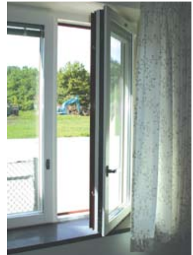
Security system window-contacts are co-utilized by the climate system
