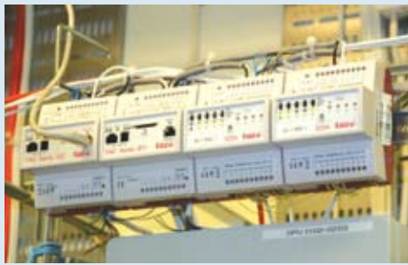
Integration and communication between climate and security systems is made possible through the Xenta 527
